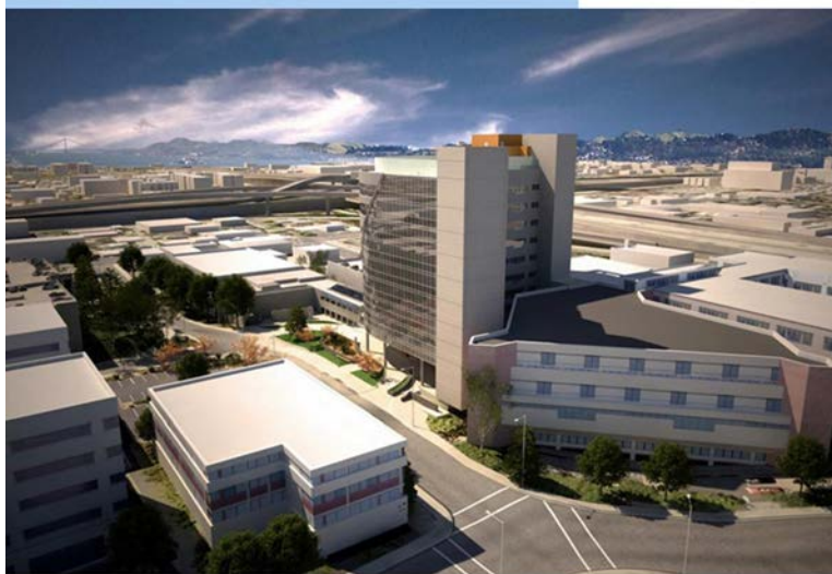
PCP tower adjacent to the existing hospital.
