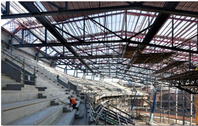
Arena during construction.
